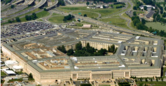
Construction Management Washington Headquarters Services Arlington, Virginia
